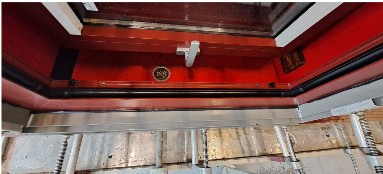
Photog. 1. View of the handle, frame drainage and locking points
