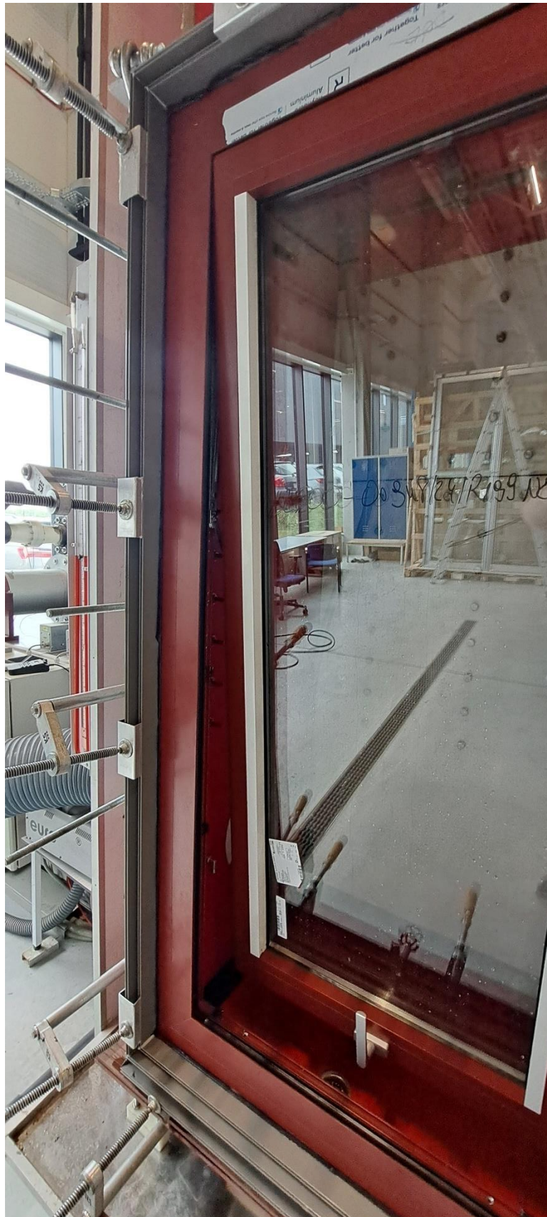
Photog. 3. View of the door in open position
